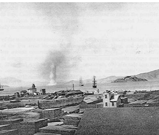
Historic photo of rock blasting to remove navigational hazards inside the Golden Gate.
